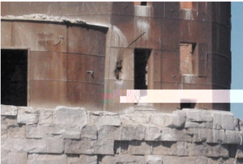
Inspection of the armor plating reveals an indentation about the same size as the partially deformed bomb in the water nearby.
